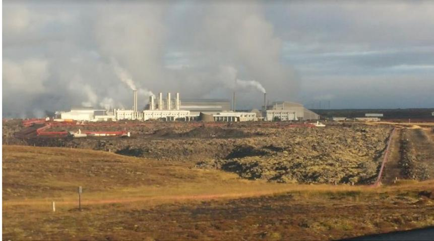
Svartsengi power station has a production capacity of 75 MW of electricity and 190 MW of heat. The PULSE™ handles water supply, electricity generation, and high voltage switching. The servers communicate with Programmable Logic Controllers (PLCs) controlling the systems that absorb steam coming from deep geothermal wells deep within the earth. Dry steam is separated for turbines generating hot water for use by residents in neighboring cities.
